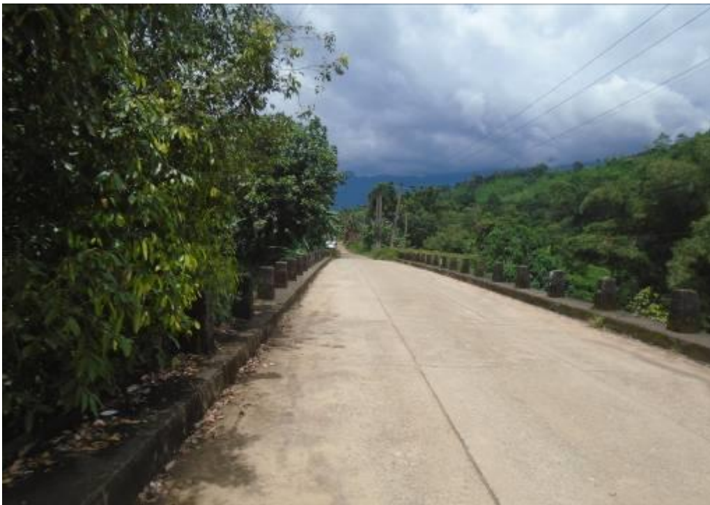
Figure 2: River crossing at 0.1km
