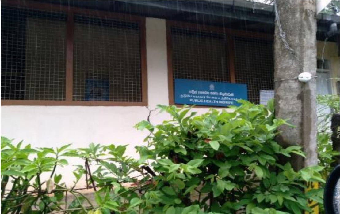
Figure 4: Public Health Centre located at 1.100km on LHS of the road
