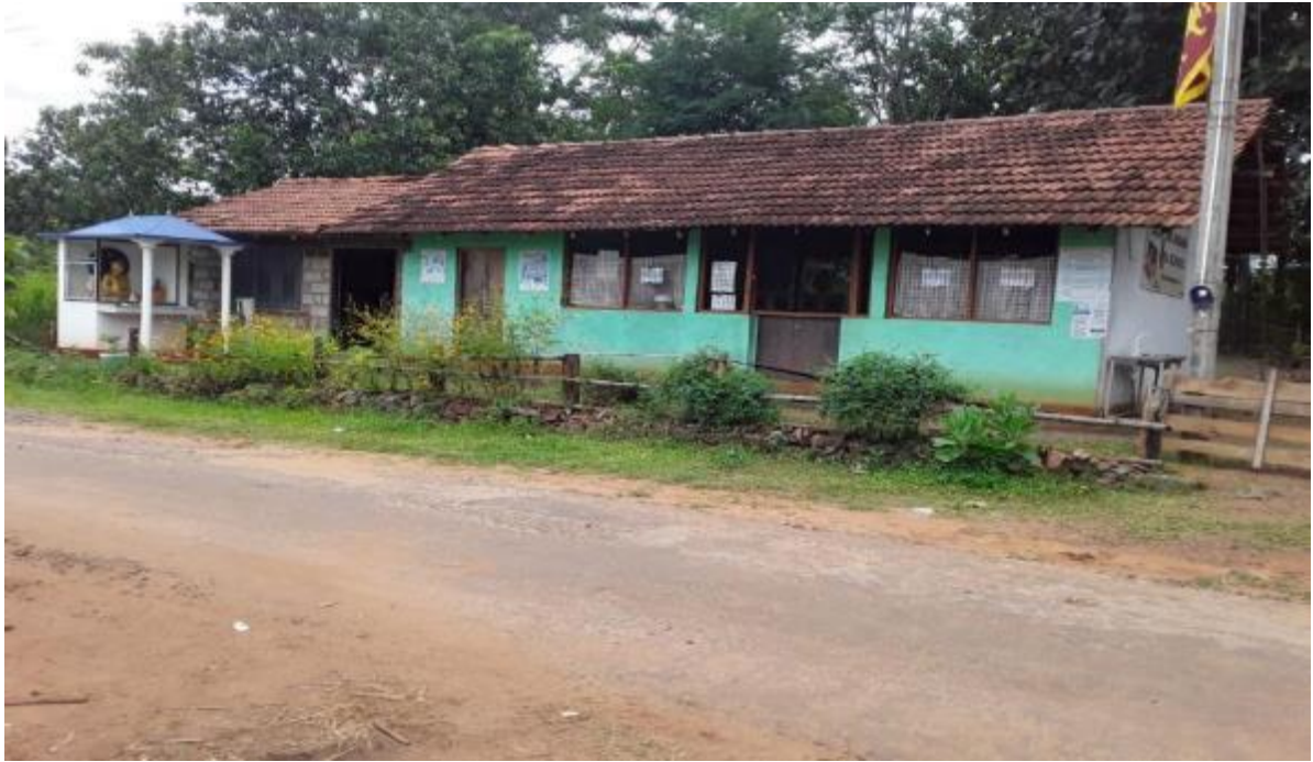
Figure 3: Pre School located at 1.900kmon RHS of the road
