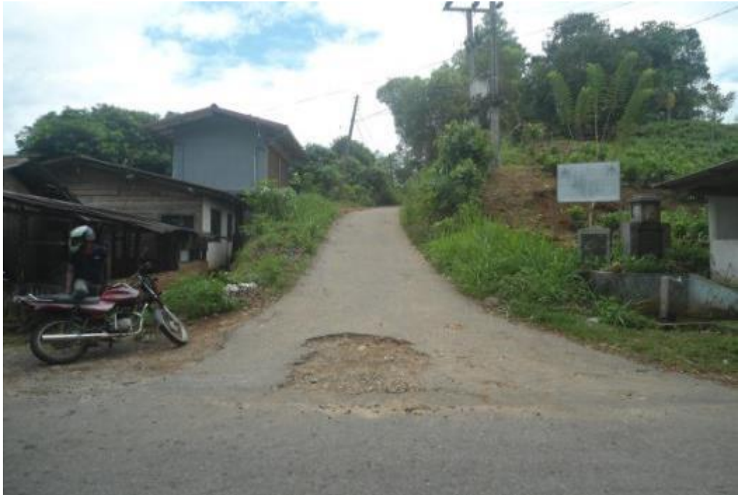
Figure 6:End point of the road
