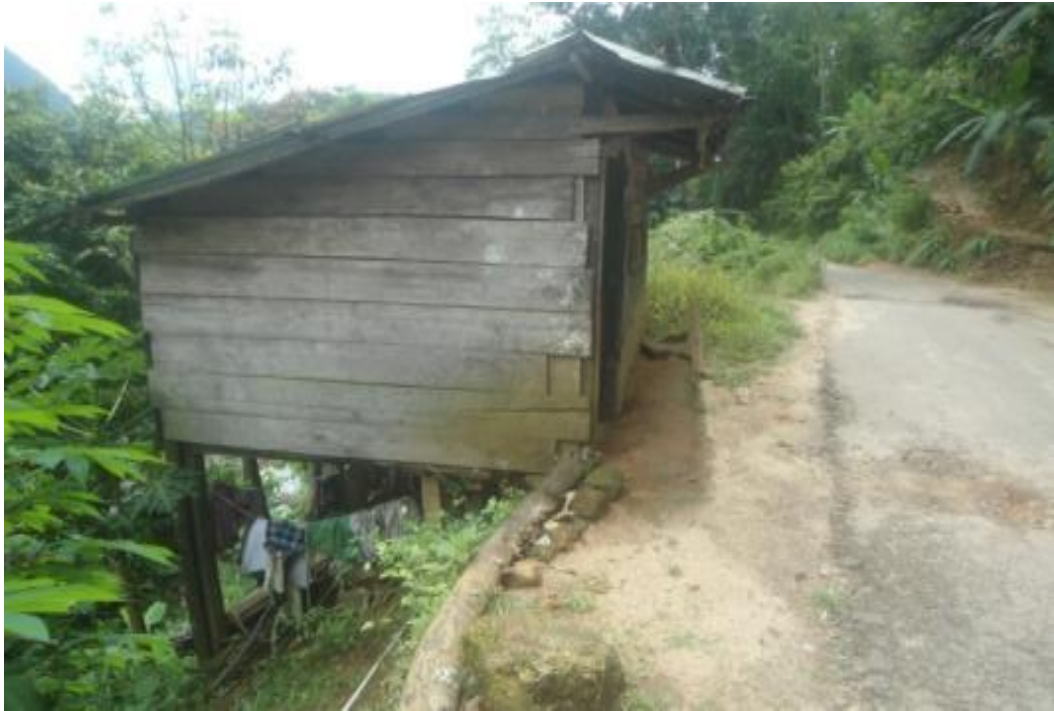
Figure 4: A squatter observed at 2.750 km on RHS of the road
