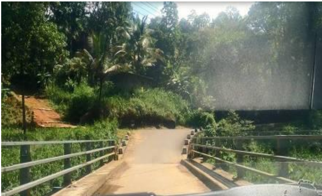
Figure 2: Stream crossing at 1.9km
