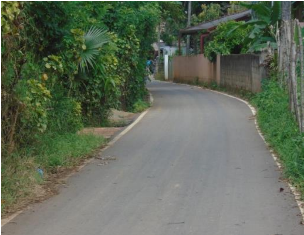
Figure 4:End point of the road
