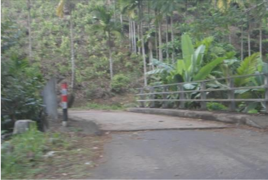
Figure 3: Bridge located at 1.350km of the road
