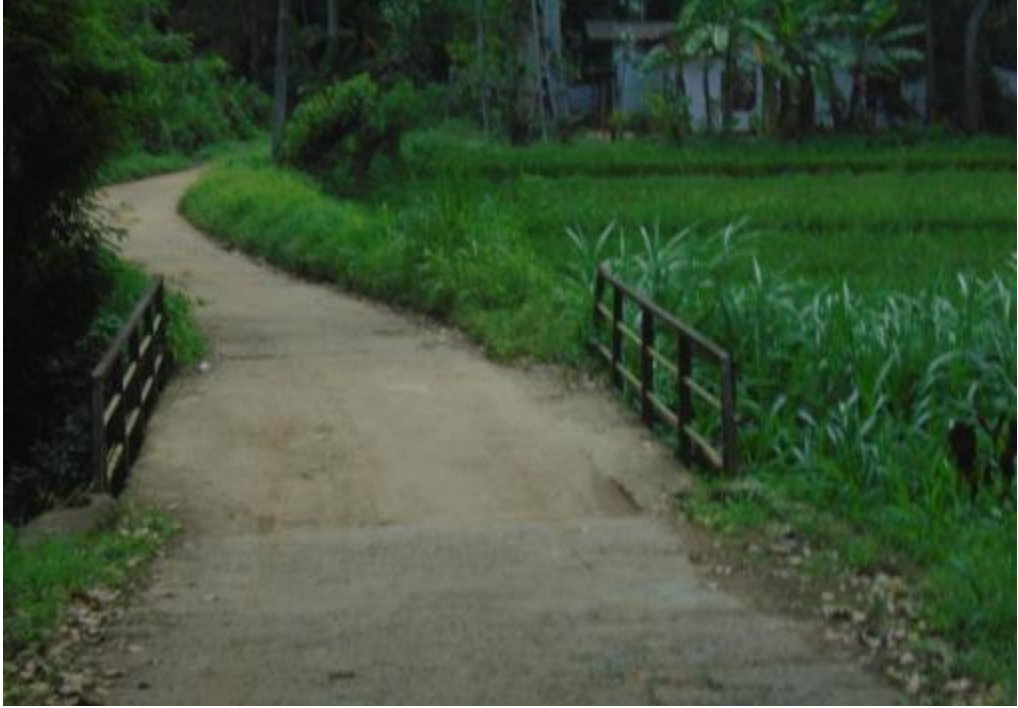
Figure 5: Bridge at 1.8 km
