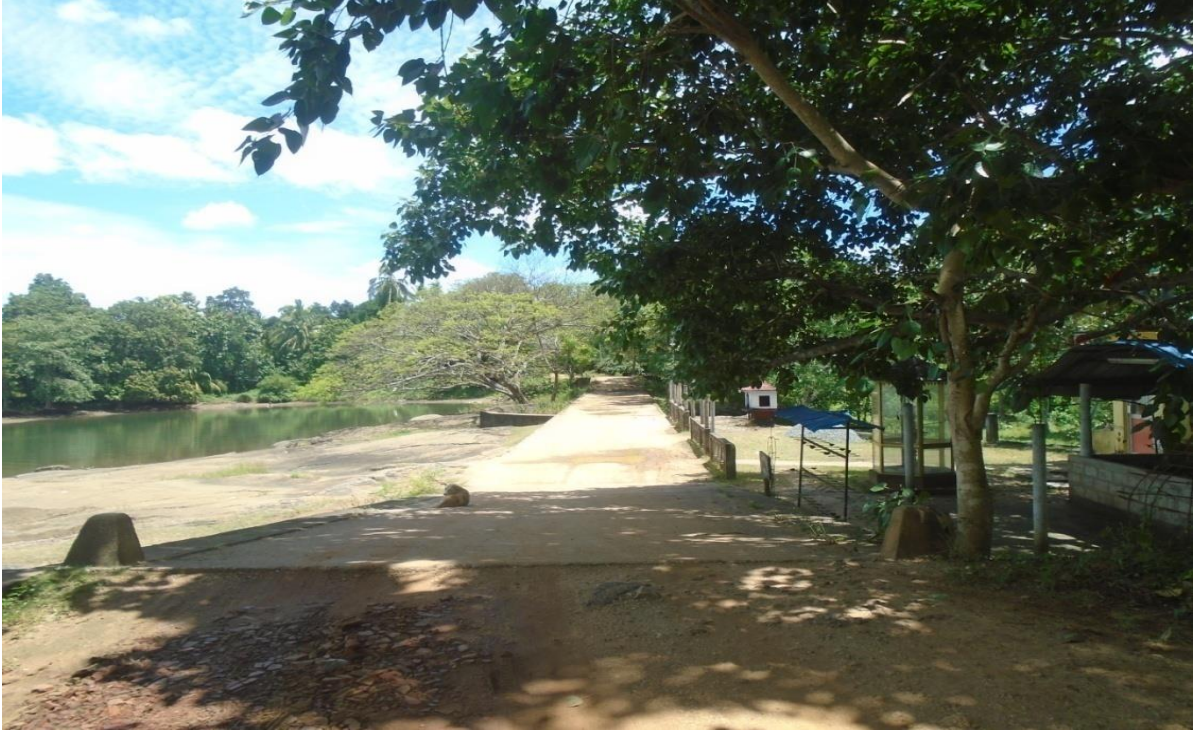
Figure 7: End point of the road
