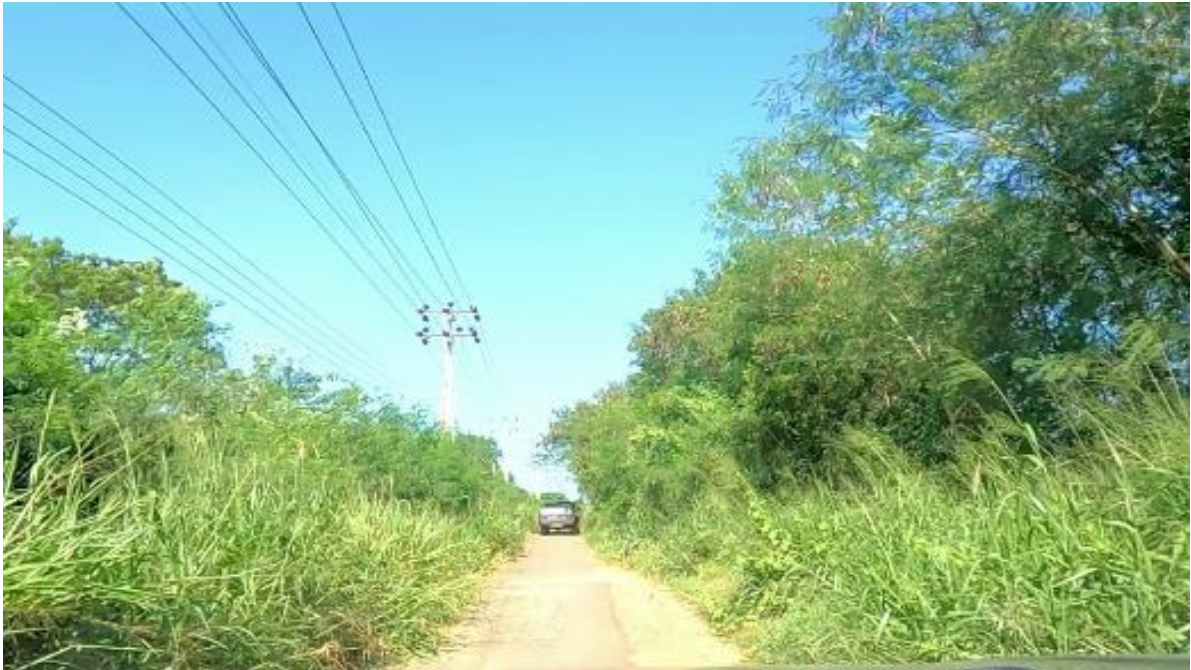
Figure 3: Gravel section of the road
