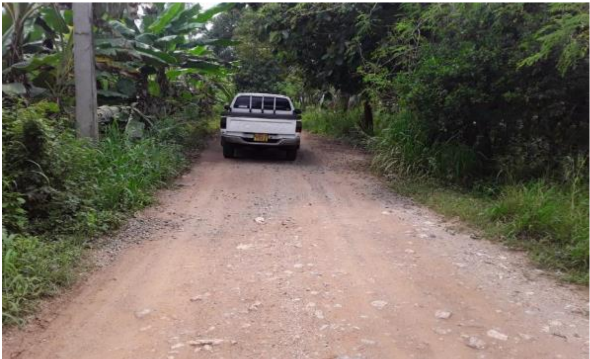
Figure 4: End point of the road
