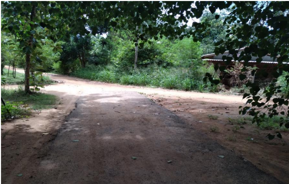
Figure 6: End point of the road
