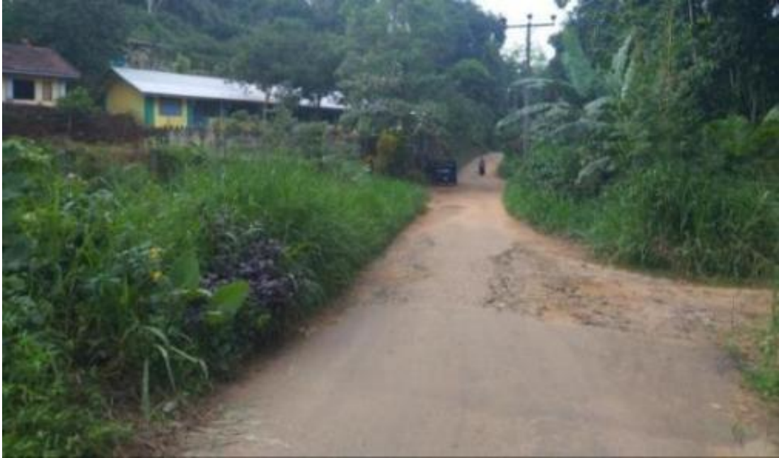
Figure 5: End point of the road
