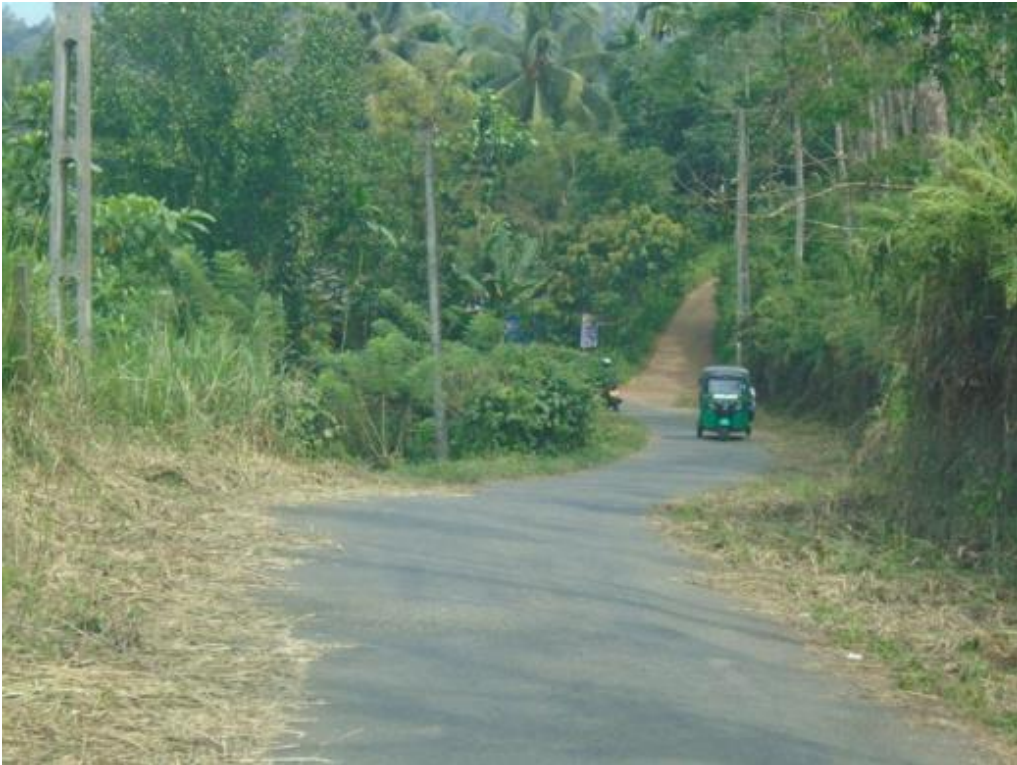
Figure 5: End point of the road
