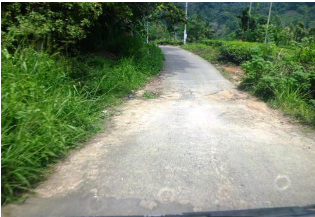
Figure 8: End point of the road at 8.0km
