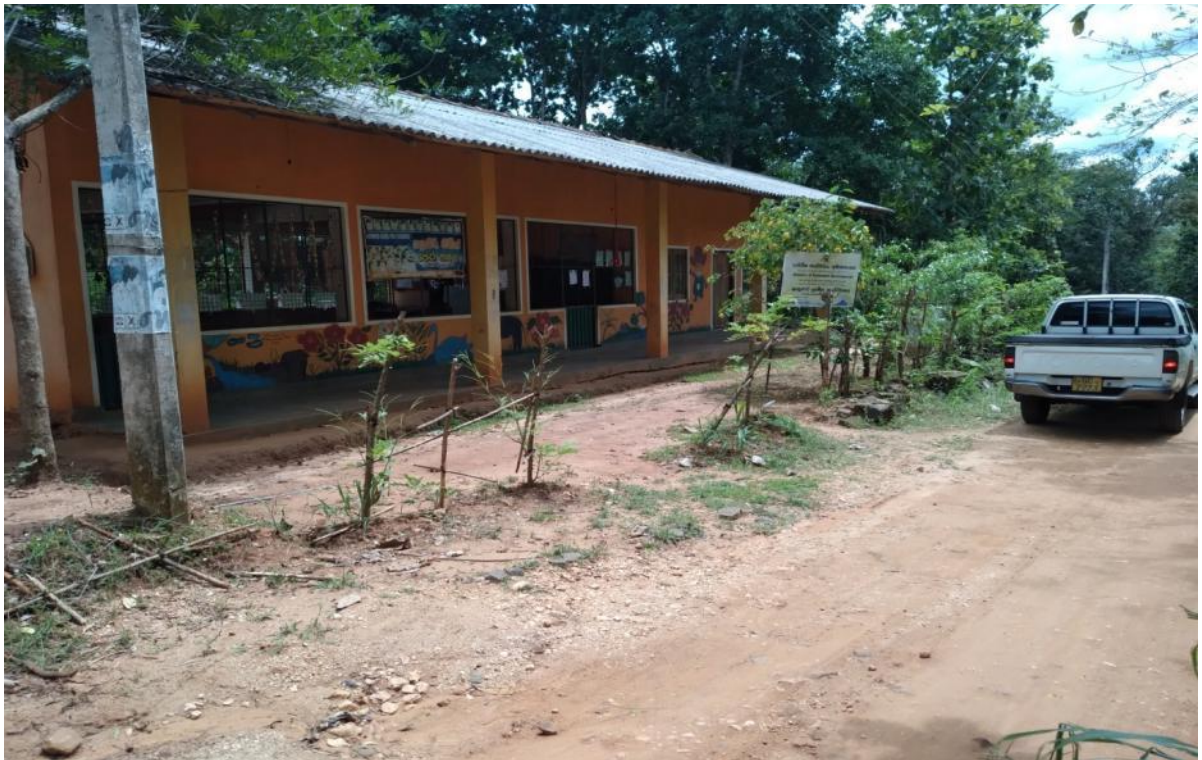
Figure 4: Pre School located at 1.080 km on LHS of the road
