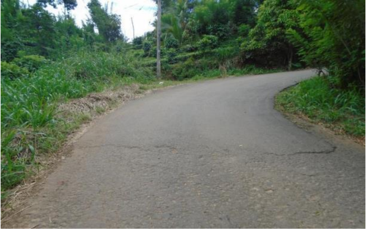
Figure 5: End point of the road
