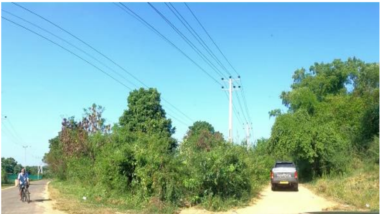
Figure 6: End point of the road
