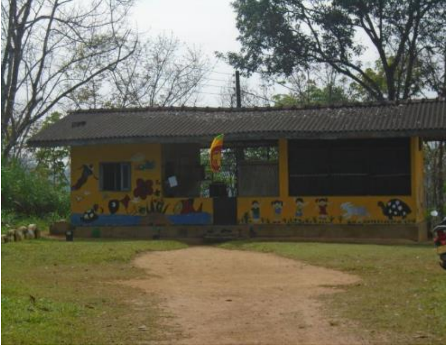
Figure 4: Preschool located at 1.260 km on RHS of the road
