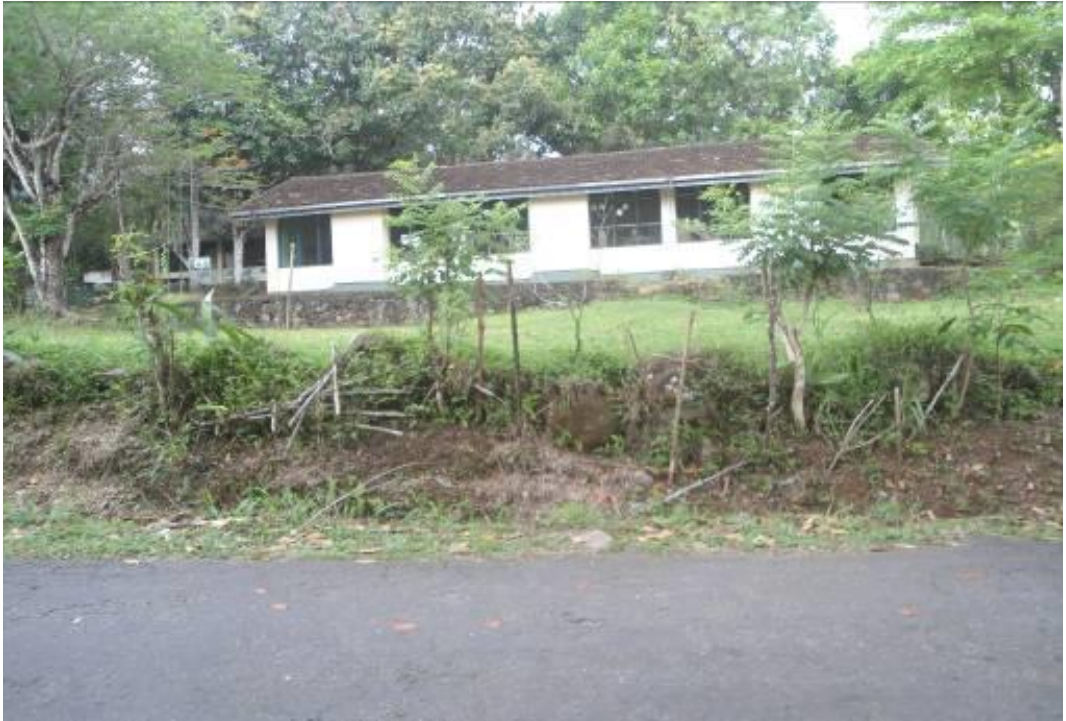
Figure 4: School located at 1.900km on RHS of the road
