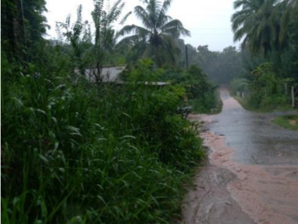
Figure 8: End point of the road
